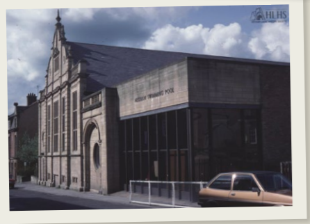
Image credits: Hexham Local History Society. 1971: Gilesgate looking E, No 13 Henry Bell wool warehouse prior to conversion to old swimming pool and demolition of adjoining buildings. 1983: Gilesgate looking N, No 13 Henry Bell wool warehouse/old swimming pool showing swimming pool extension.
